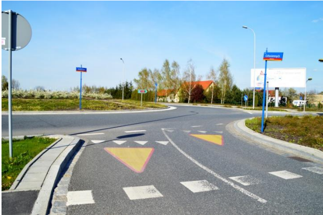
At the ringroad entrance there is a need of clearly visible marking of necessary giving way to the transport moving on the ringroad. There was used mark „Give way” at the every traffic line.
