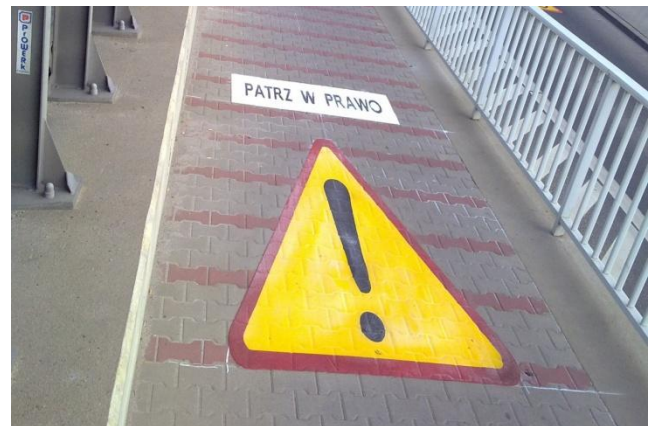
Bicycle track with limited visibility also requires special mark for cyclists. There were used an „Attention!” mark with an additional informative mark.
