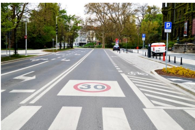
New slow moving traffic line required simple and readable mark. There were used „Limited speed zone” marks at the both sides of the traffic line.
