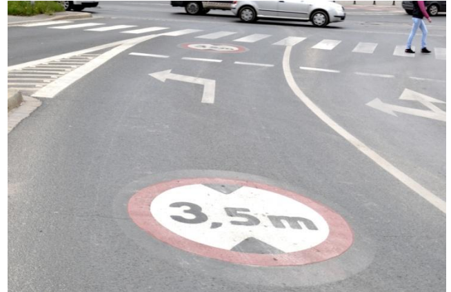
There is a need to early inform drivers about transport height allowed to move under an overpass. There was used „No vehicle over 3,5 m height” sign serie.
