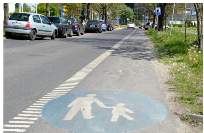
Due to lack of a sidewalk, there is allocated for pedestrians line on a road. There were used „Pedestrians-only road” marks for each 50 meters of the line.
