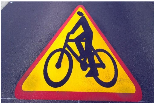
Bicycle track with limited visibility requires high contrast mark, that will draw driver's attention. There was used „Cyclists” mark serie.
